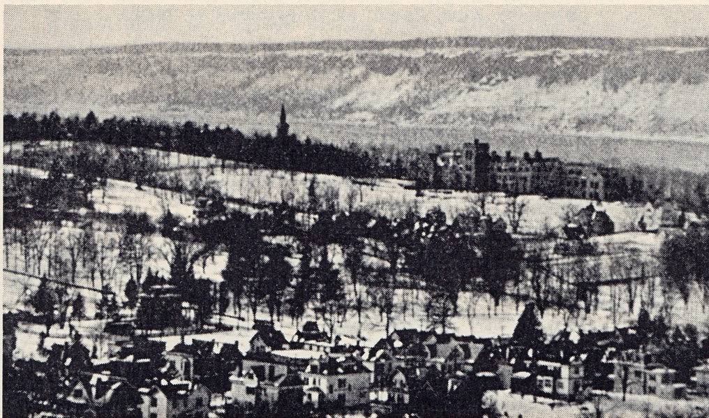
View of the Hudson as it appeared from the hotel site on Park Hill in the early 1900s.
